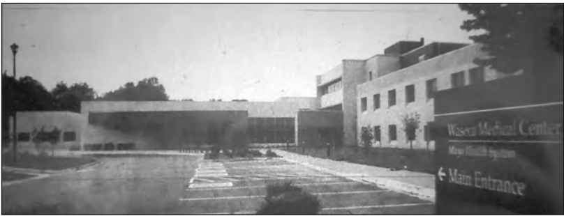
-Pictured is the new entrance to the Waseca Medical Center. The public is invited to see the results of the 10-month construction project on Sunday, September 12 from 1 p.m. to 4 p.m. There will be refreshments, prizes, tours and a very short program at 2 p.m.
