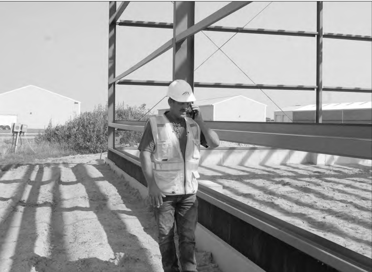
Mark Indrelie of Mankato-based construction company APX, is overseeing the construction of the new hangar at the Waseca Municipal Airport. Pioneer photo by Ben Revermann
