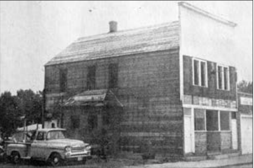
- A 60 foot by 70 foot fire hall containing not only room for the Waldorf Volunteer fire department's trucks, but also a meeting room, restrooms and kitchen will be erected on the lot in Waldorf, where the old village liquor store building is being dismantled, soon. A call for bids appears in this issue of the Star. Residents of the village voted 74 for the issuance of $45,000 bonds and 16 were against at the special election, Monday.
