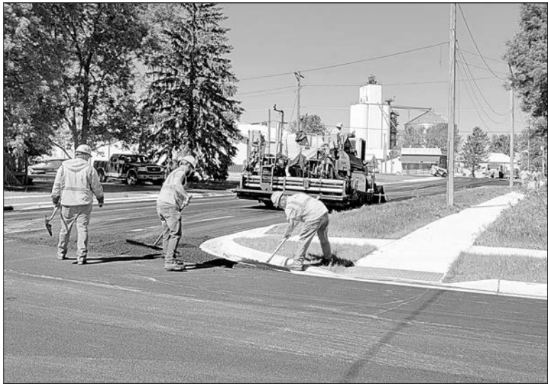
Judy Joecks of Waldorf snapped some neat photos of the street crewing laying new roads in town, shown above.
