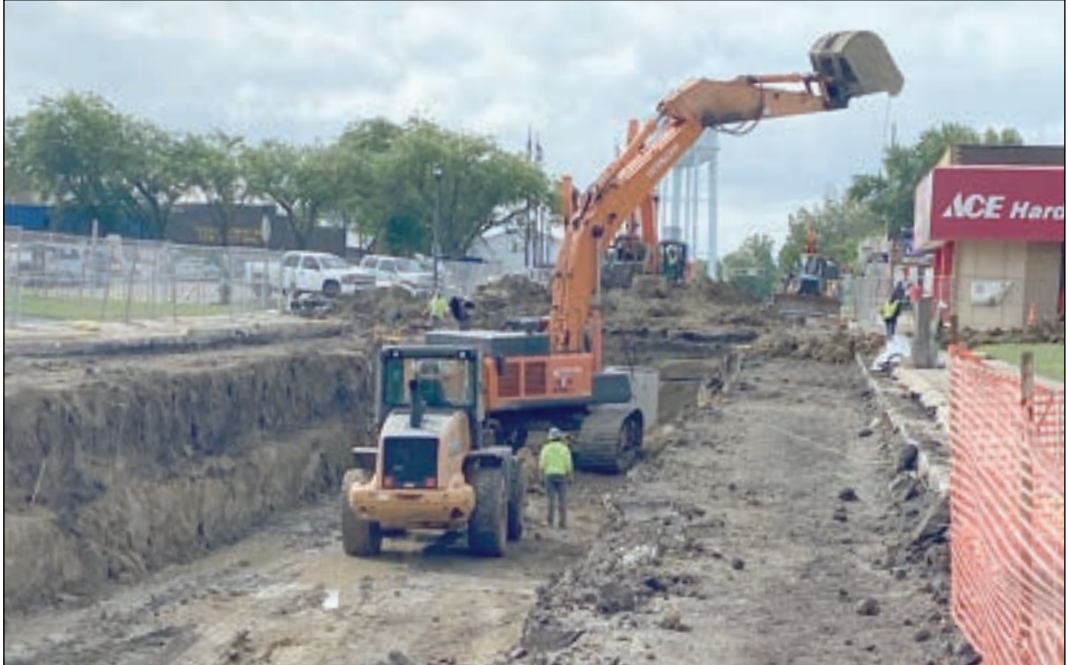
ONGOING WORK - Construction continues on Second Street in Waseca, causing difficult access to businesses like the Waseca Area Neighborhood Service Center and Waseca Area Food Shelf. Pioneer photo by Deb Bently
