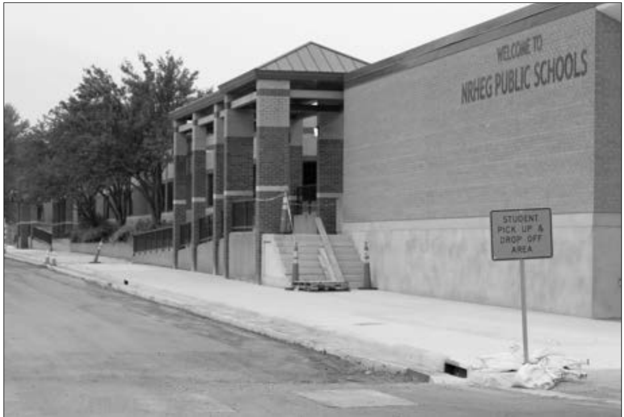
ROUTE CHANGE - As the school year begins, unfinished construction is causing some complications for transportation. Until the usual route is suitable for traffic, buses will be turning around and driving back north on South Ash Avenue. Parents dropping off students are asked to drive through the parking lot to return to Highway 30.
