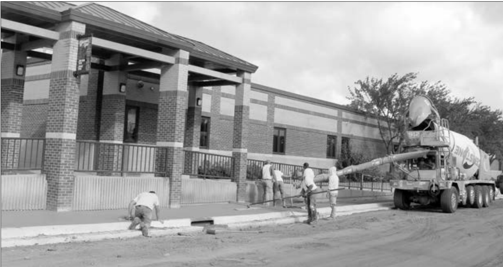
COMPLICATIONS - Ongoing construction will interfere slightly with operations as the NRHEG school year begins. Street work which was scheduled to be complete before September was delayed by this year's rainfall. Here, a construction crew put in time on a recent Saturday to pour and level cement on sidewalks. Pioneer photo by Deb Bently
