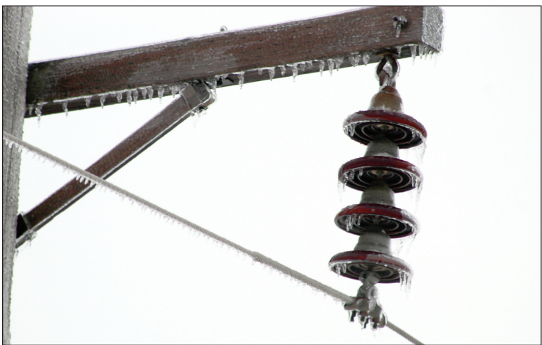
An iced over powerpole, insulator, and powerline outside New Richland during this week's ice storm. Pioneer photo by Deb Bently
