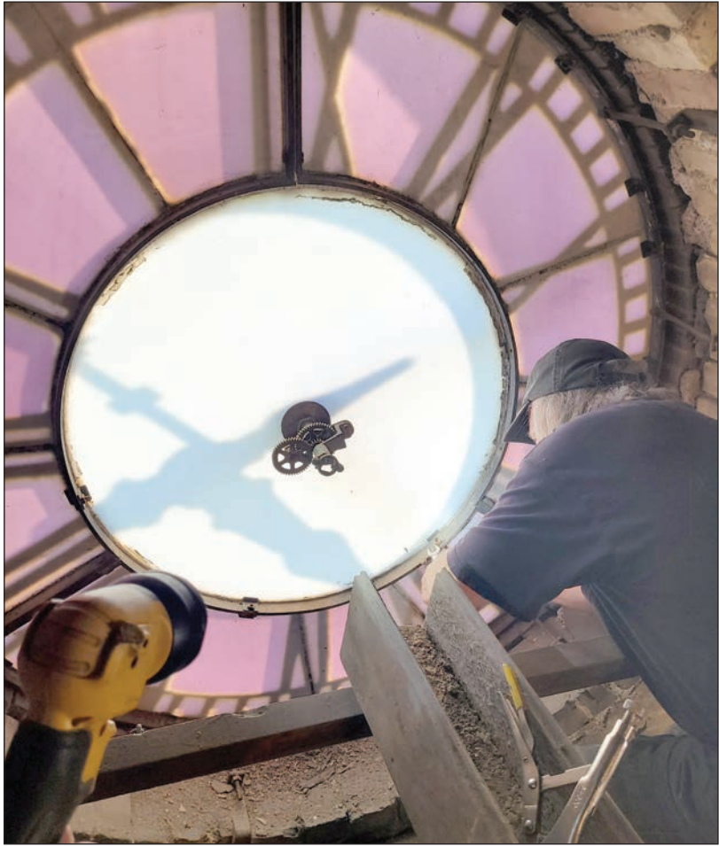
Waseca County facilities director Brian Tomford examines one of the courthouse clock faces from behind during some maintenance work. Made of a special type of glass called "vitrolite," the faces are between five and six feet across.
