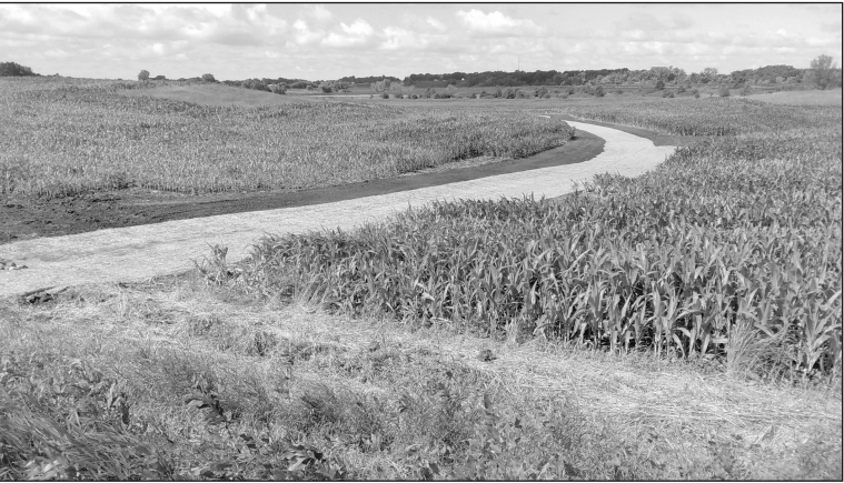
Image displays a newly completed grass waterway that was built with the assistance of Waseca SWCD.
