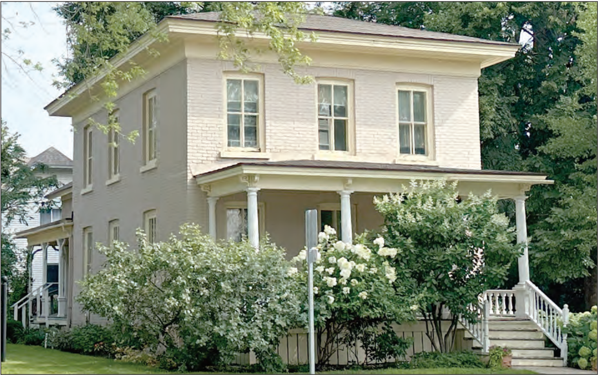
MERCHANT HOUSE - Built in 1868, the historic Bailey-Lewer house at 401 Second Avenue Northeast in Waseca, is the oldest existing house within Waseca County. Structural problems have officials studying the best way to facilitate upgrades.
