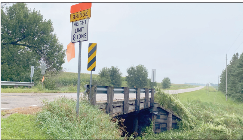
This bridge along County Road 6 northeast of New Richland was built in 1940. Stress tests showed it is no longer safe for vehicles over 8 tons. Originally scheduled for replacement in 2027, it will now be replaced in the next few months. Pioneer photo by Deb Bently
