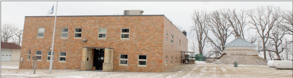
Under plans for expansion and improvement, the Waterville Fish Hatchery’s original block structure will remain and be remodeled. Another building will be added to the grounds.
