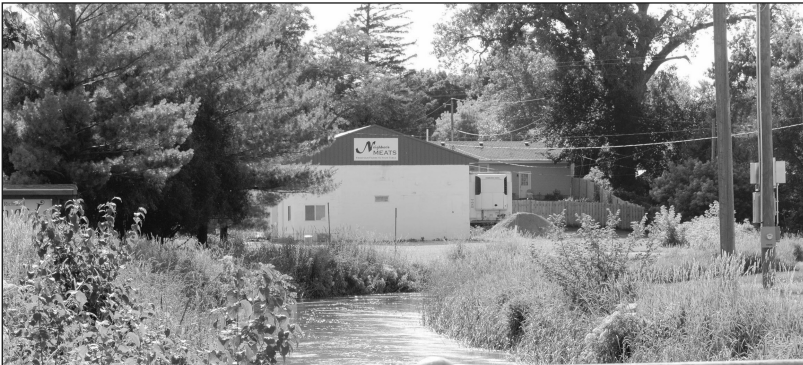
Wastewater from New Richland's water treatment system had to be diverted into Boot Creek, which runs through the town.
