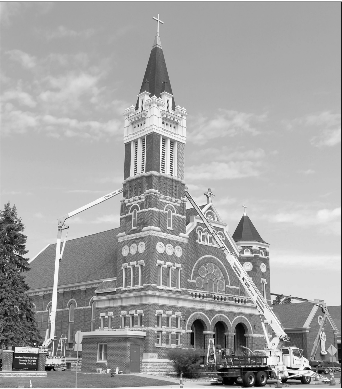
Workers from Krause Konstruktion of Coon Rapids, Wisconsin, will spend about three weeks finding and replacing patches of mortar on the walls and tower of Sacred Heart Church in Waseca. Pioneer photos by Deb Bently
