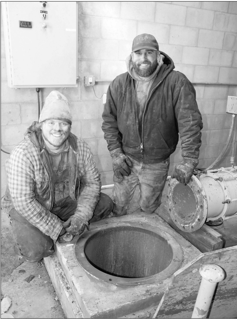
The start of the maintenance process for each of the city's wells is to remove the metal shaft which houses the pump. Here, two workmen have finished using a derrick to remove hundreds of feet of pipe and are next to the open well, which extends nearly 1,000 feet underground.
