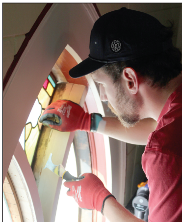
Cathedral Crafts craftsman Neil Callahan installs a window at North Waseca Lutheran Church.
