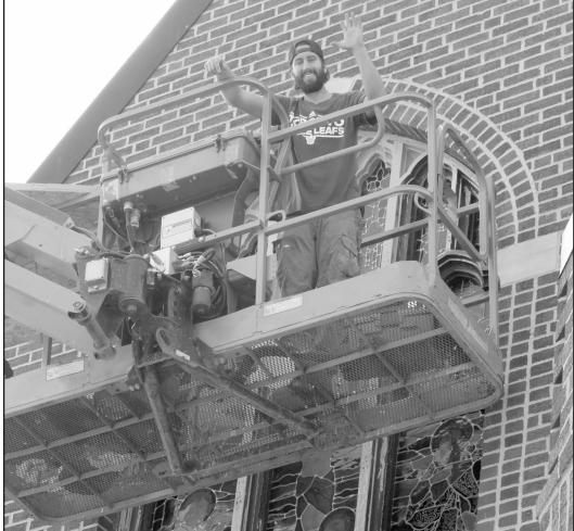
FINAL STEP - Caleb Penic of Winona's Cathedral Crafts previously worked on All Saints Catholic Church's windows in 2018. Photo by Deb Bently
