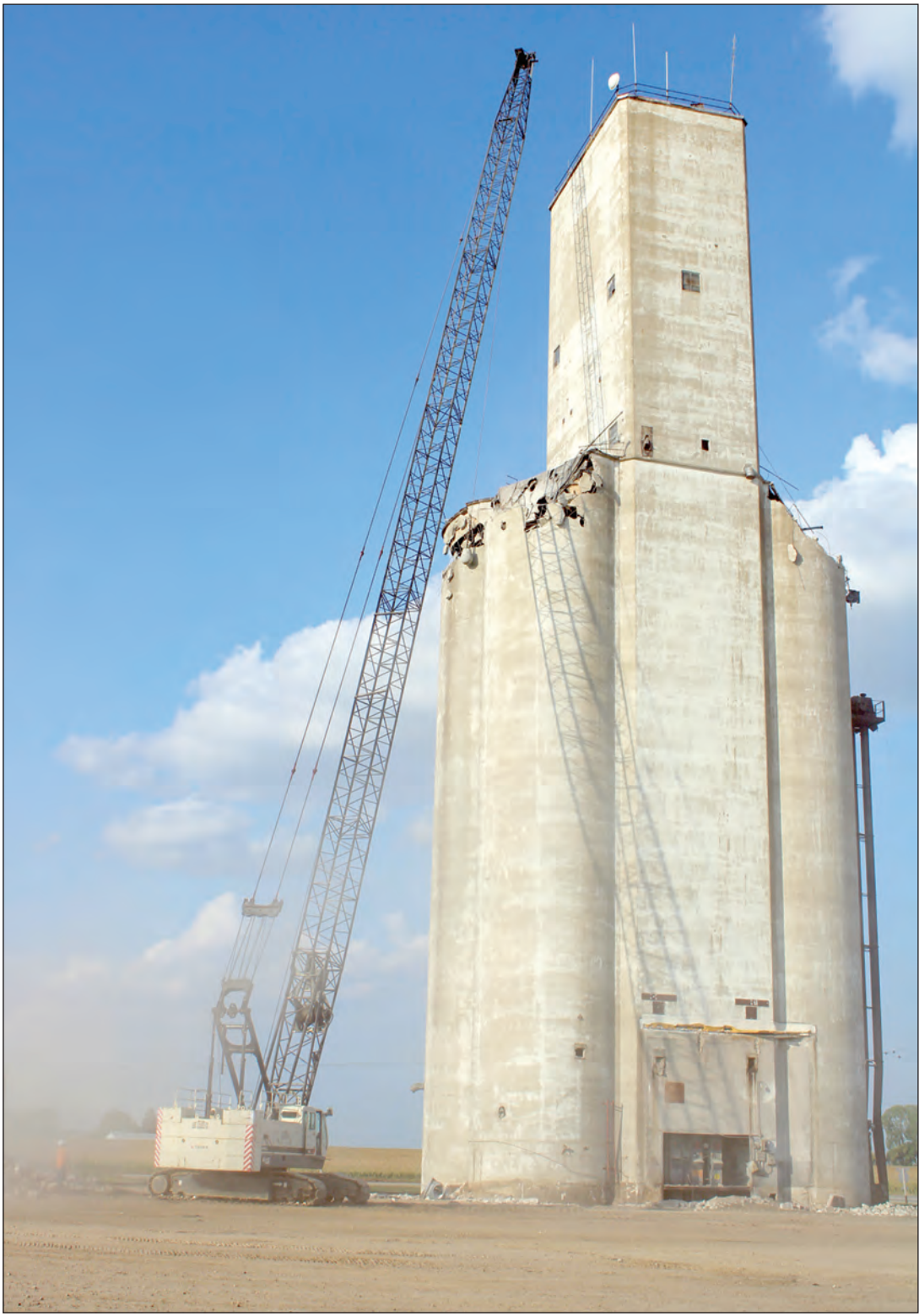
A 150-foot-tall crane swings a wrecking ball against one of the structures at Crystal Valley Coop between Janesville and Waseca. Pioneer photo by Deb Bently
