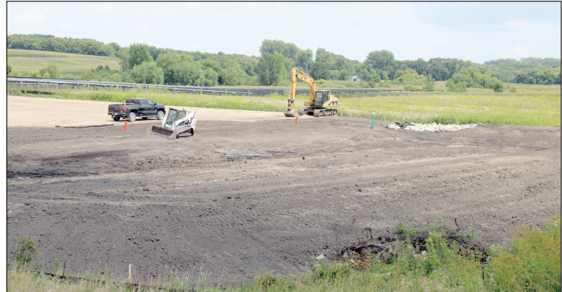
UNDER CONSTRUCTION - Equipment from Evans Companies Landscaping of Byron finishes construction on the new composting site.
