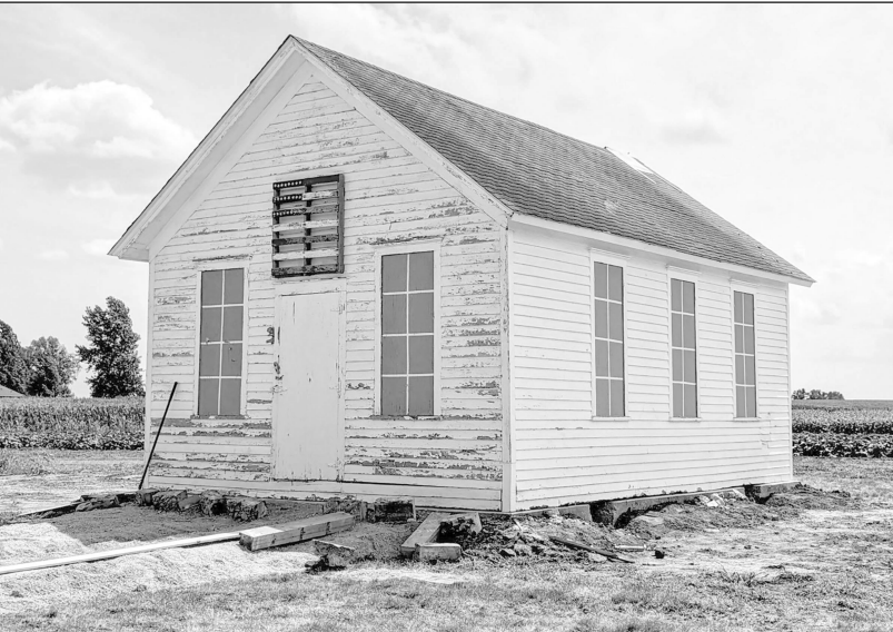
IN PLACE - Over the next months, the Autumn Acres schoolhouse will be renovated for use on the farm. Submitted photos
